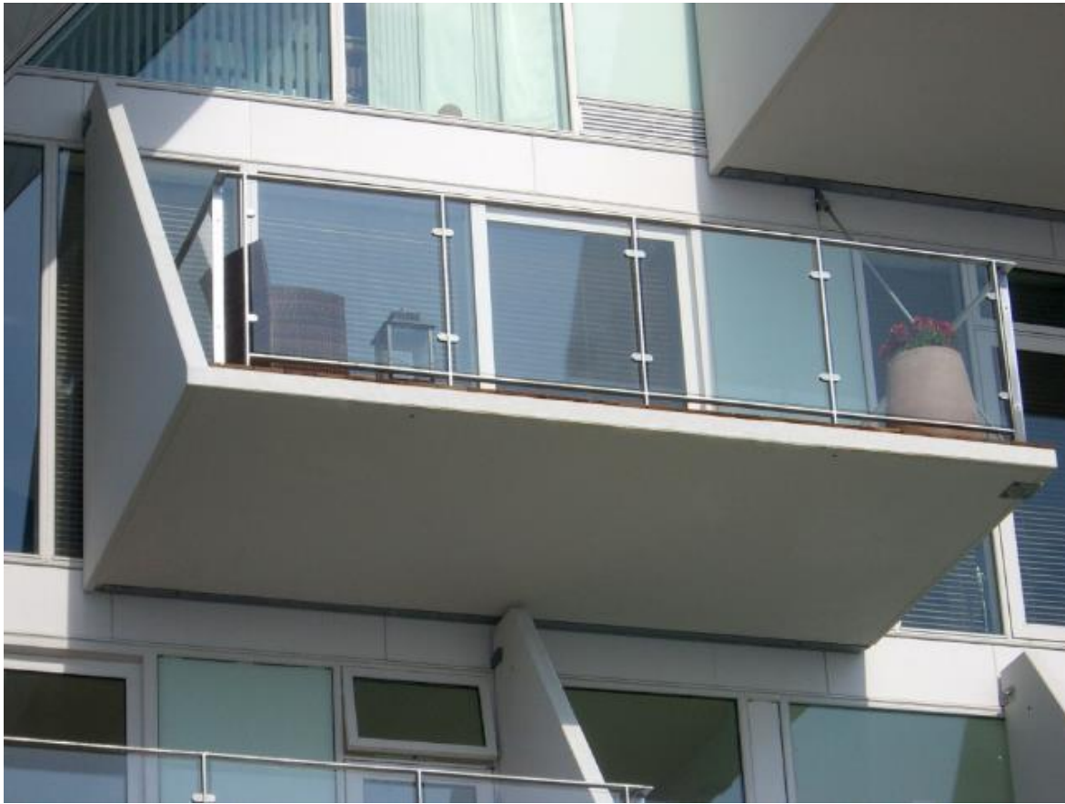
Fig. 6 Balcony combining concrete upstand and strut.
