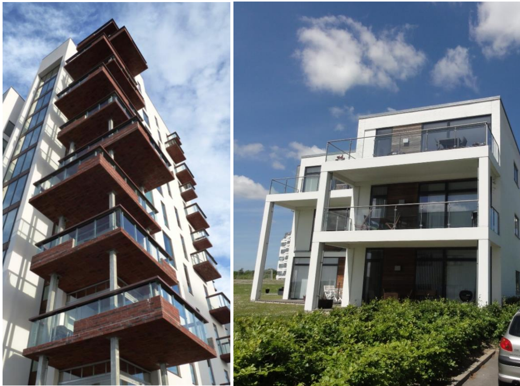
Fig. 3: a) Balcony elements partly supported by columns. b) The outer edge of the balcony element contains an integrated beam/rib.
