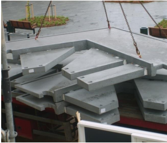
Figure 1: Cantilevered balcony elements ready for installation. The cantilevered flaps are cast monolithically as part of the element for attachment to the building façade.
