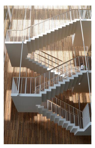
Type of staircase: Accordion staircase
