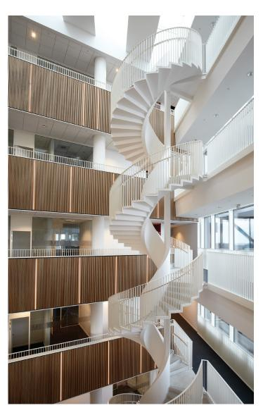
Type of staircase: Winding staircase
